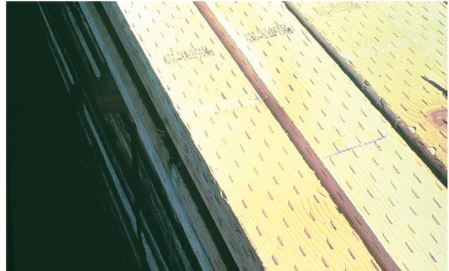
Figure 2. Incised lumber to improve the penetration of the treatment chemical.
