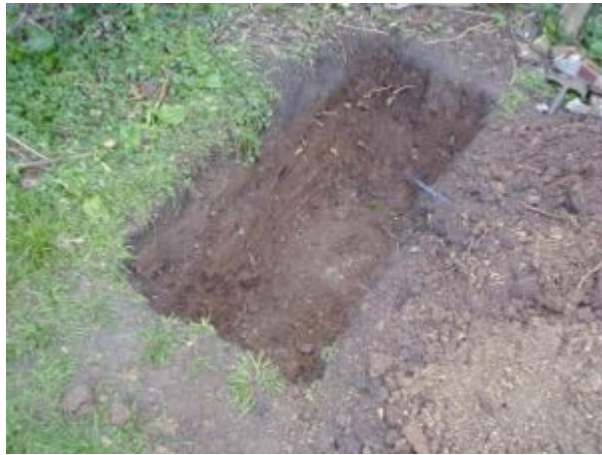
A Small test block and 1.5 meter deep hole partially finished for the test block.
